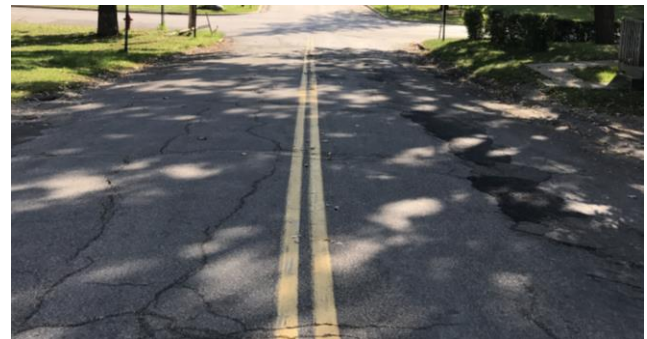
Existing Pavement Conditions
